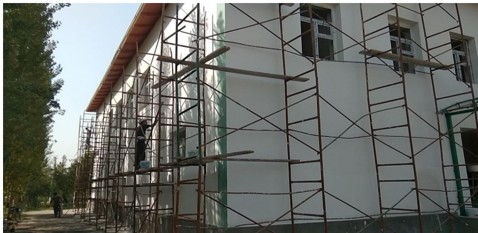
Campus №7. Maintenance work August, 2023
