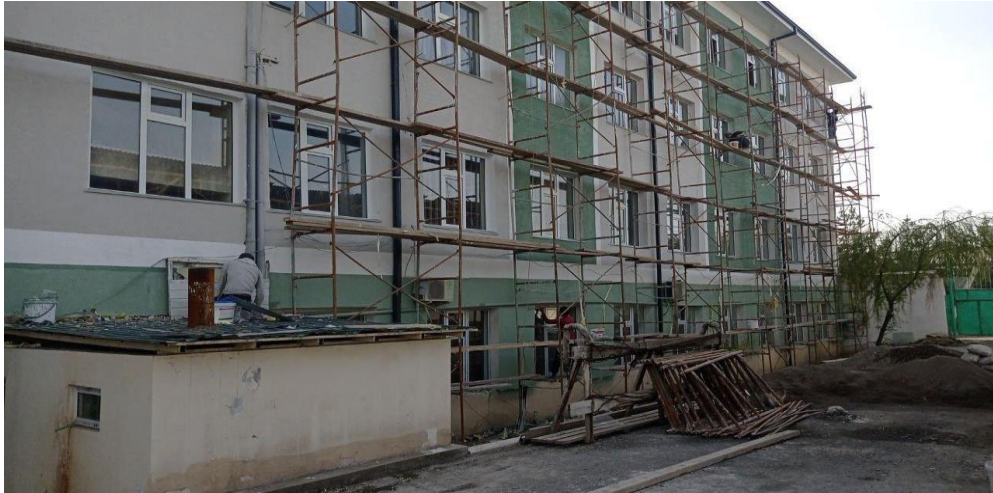
Campus № 4. Maintenance work August, 2023
