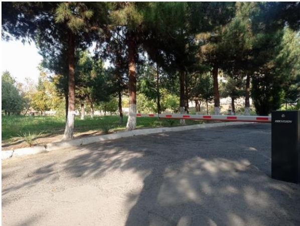
7. automatic barrier gate
