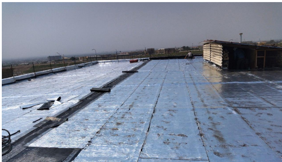
Maintenance of main campus rooftop (Namangan Engineering-Construction Institute) August, 2023
