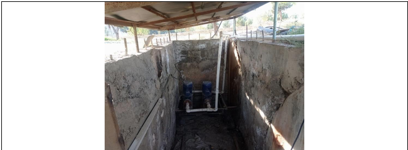
Example of Sewage Disposal (Namangan Engineering-Construction Institute (NameCI))
