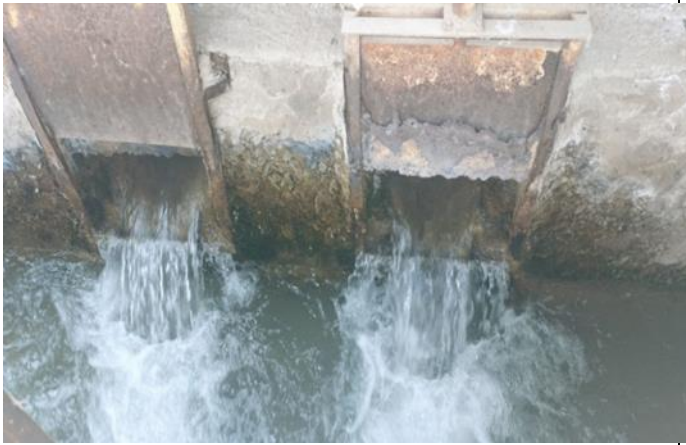
4. Kyzilrovot drinking water treatment plant
